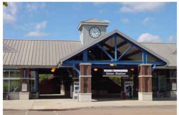
Union Station at entrance of campus
